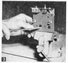
Held firmly in a bench vise, the perforated Bakelite board is easily drilled and cut to shape desired.
